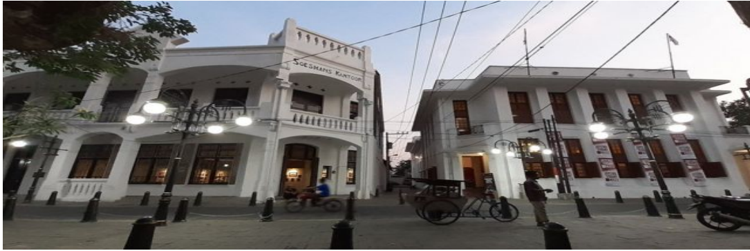
The Huis Monod Building (right), a relic of the Dutch colonial era, has been restored.
