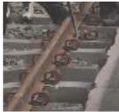
Gambar 2.20 Penambat Rel Spring Clip.
