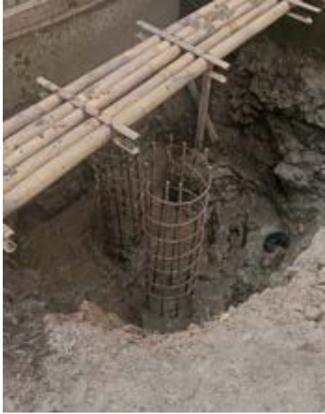
Gambar 4.14 Tulangan Bore Pile
