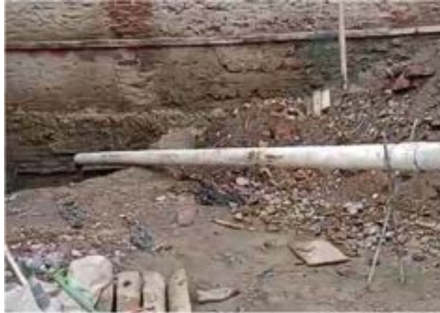
Gambar 4.15 Pengecoran Lubang Bore Pile
